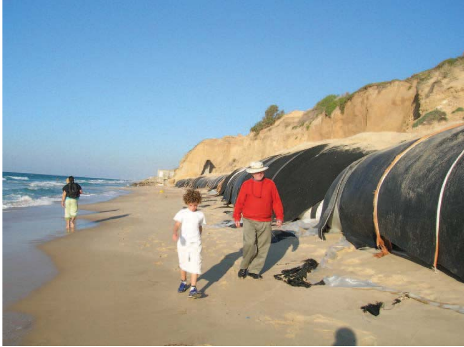
Figure 8. A temporary coastal protection at Ashkelon Mayumas using a geo-technique sleeve filled with sand (E Galili).
