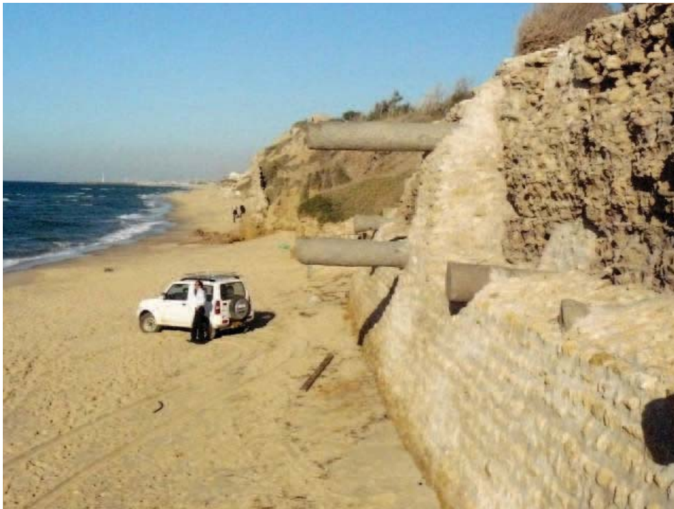
Figure 3. The Ashkelon seawall after conservation (E Galili).
